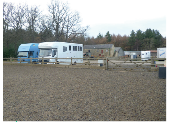
Parking and public areas should be well away from the main yard.
