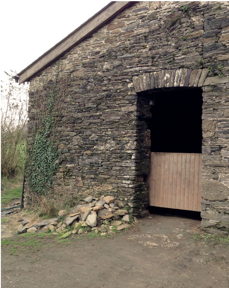
Ideally the isolation area should be in a separate building.
